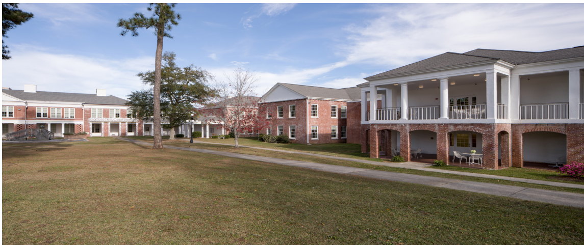
Roosevelt Warm Springs Health Facility Improvements, Photo courtesy of Barton Malow Company © Jason Buch Photography
