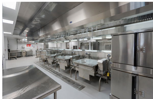
Metro State Prison, Science and Technology Facilities Photos courtesy of Wakefield Beasley & Associates
