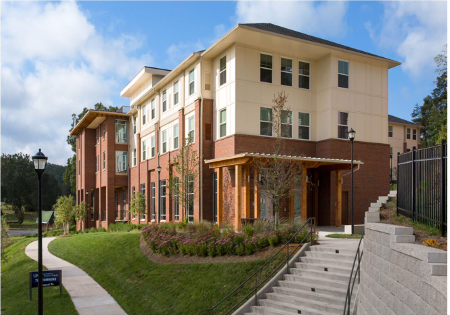
University of North Georgia – The Commons Dahlonega, Georgia Submitted by the Board of Regents
