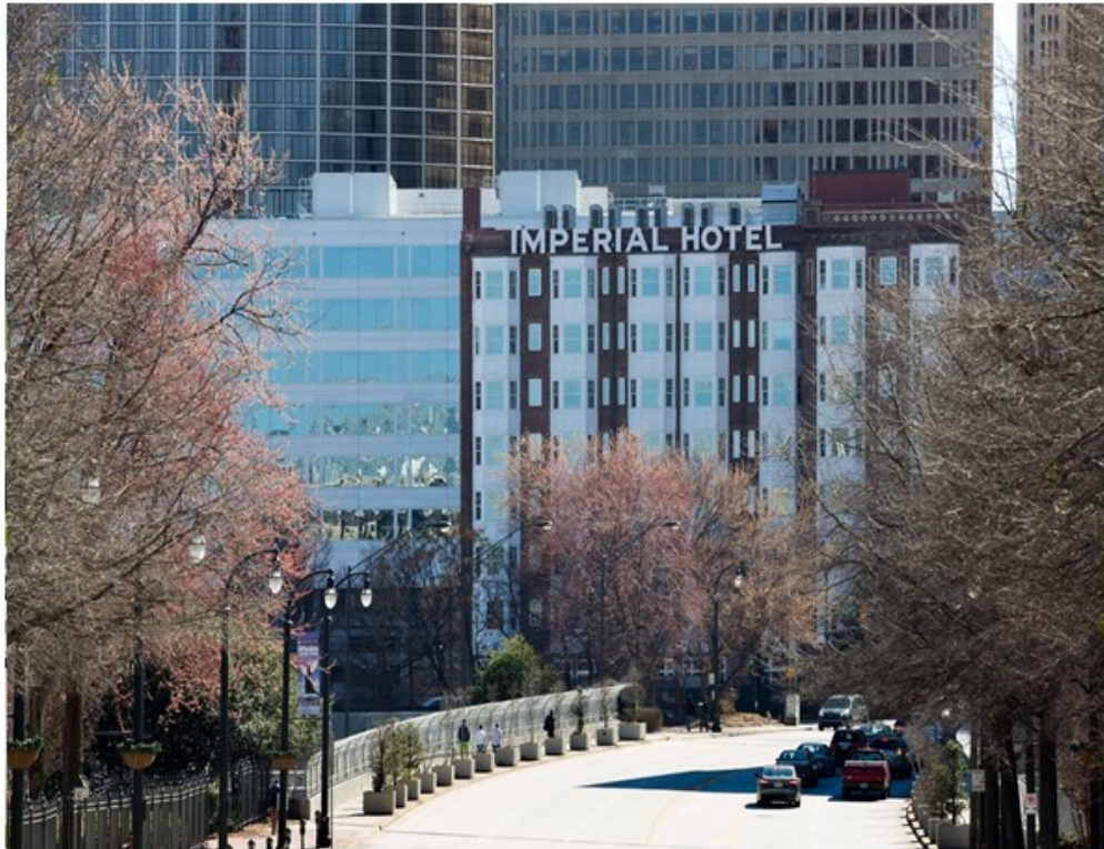
Imperial Hotel – LIHTC AND HOME Programs Atlanta, GA Submitted by the Department of Community Affairs
